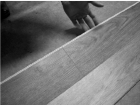
Fig. 6 - Locking long side with ends already locked
