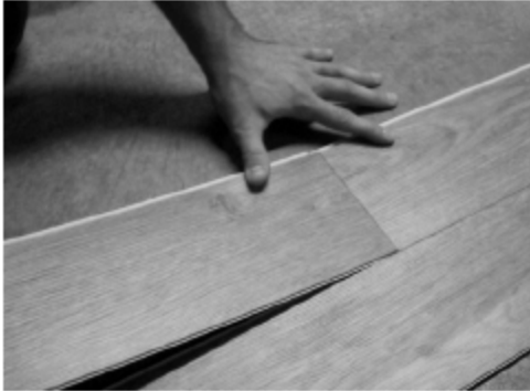
Fig. 5 - Angle end of next plank
