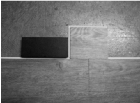
Fig. 7 - Tap side of plank with tapping block
