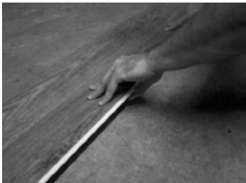
Fig. 4 - Angle long side into prior row.
