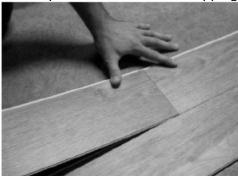
Fig. 4 – Angle end of next plank
