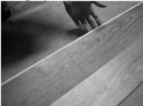
Fig. 5 – Locking long side with ends already locked
