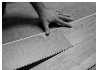
Fig. 5 – Angle end of next plank.
