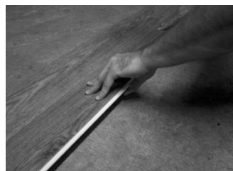
Fig. 4 – Angle long side into prior row.
