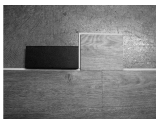
Fig. 7 – Tap side of plank with tapping block.
