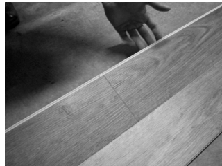
Fig. 6 – Locking long side with ends already locked.
