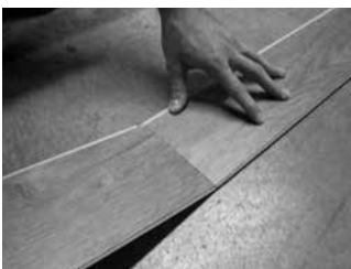
Fig. 3 – Angle end tongue into end groove on planks in the initial row.
