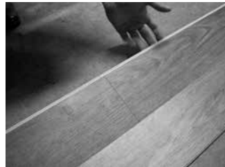
Fig. 6 – Locking long side with ends already locked.
