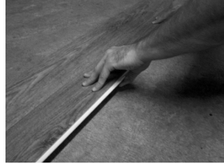
Fig. 4 – Angle long side into prior row.
