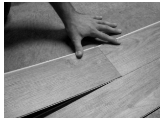
Fig. 5 – Angle end of next plank.
