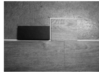
Fig. 7 – Tap side of plank with tapping block.
