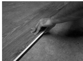
Fig. 4 – Angle long side into prior row.
