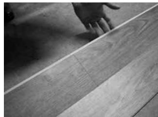
Fig. 6 – Locking long side with ends already locked.
