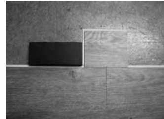
Fig. 7 – Tap side of plank with tapping block.
