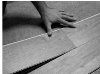
Fig. 5 – Angle end of next plank.
