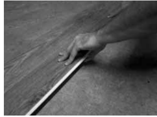
Fig. 4 – Angle long side into prior row.
