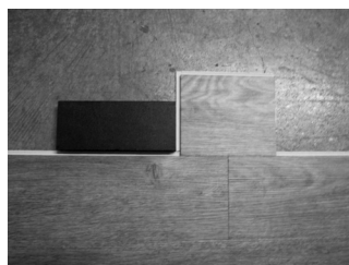
Fig. 7 – Tap side of plank with tapping block.
