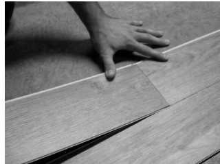
Fig. 5 – Angle end of next plank.
