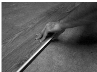
Fig. 4 – Angle long side into prior row.
