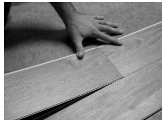
Fig. 5 – Angle end of next plank.
