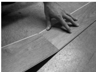
Fig. 3 – Angle end tongue into end groove on planks in the initial row.
