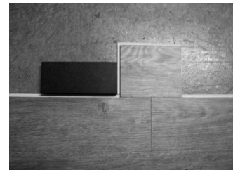
Fig. 7 – Tap side of plank with tapping block.
