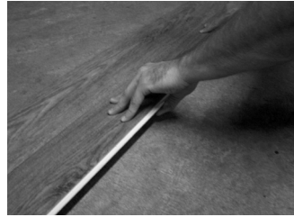
Fig. 4 – Angle long side into prior row.
