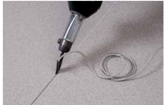
Weld rod seam
