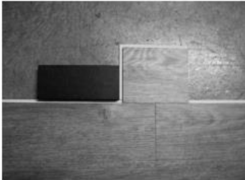
Fig. 7 - Tap side of plank with tapping block
