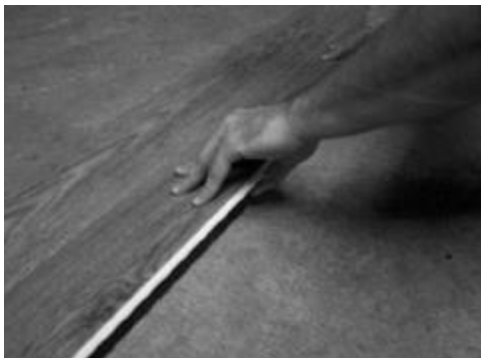
Fig. 4 - Angle long side into prior row.
