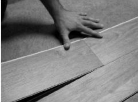
Fig. 5 - Angle end of next plank
