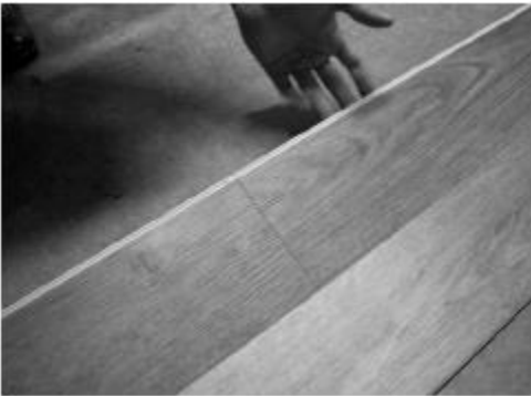
Fig. 6 - Locking long side with ends already locked
