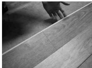
Fig. 6 – Locking long side with ends already locked.
