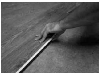
Fig. 4 – Angle long side into prior row.
