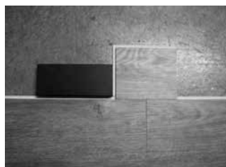
Fig. 7 – Tap side of plank with tapping block.
