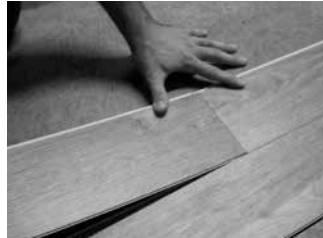
Fig. 5 – Angle end of next plank.
