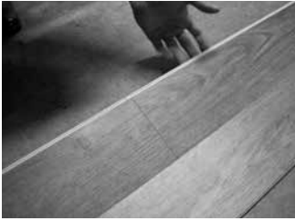
Fig. 6 - Locking long side with ends already locked
