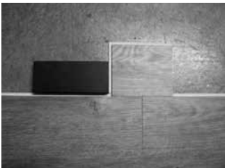
Fig. 7 - Tap side of plank with tapping block
