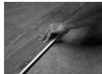
Fig. 4 - Angle long side into prior row.
