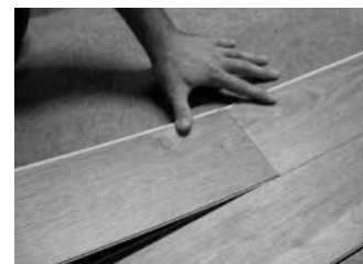
Fig. 5 - Angle end of next plank
