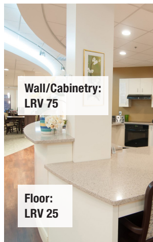
Photograph 2: LRV is used to create appropriate contrast between surfaces. Thirty (30) points minimum difference in LRV between a horizontal surface and a vertical surface provides appropriate contrast.
